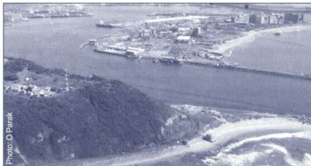
Durban's harbour is a site of stormwater discharge
